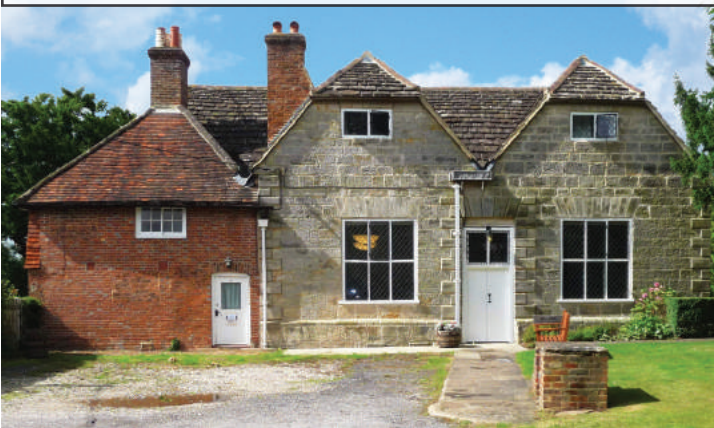
Figure 3. Southwest façade of the Friends Meeting House in Ifield, a neighborhood in the Borough of Crawley, West Sussex (1675–76), built next to an earlier residence in brick (at the left). Photo: Basil Jradeh, Wikipedia Commons.
