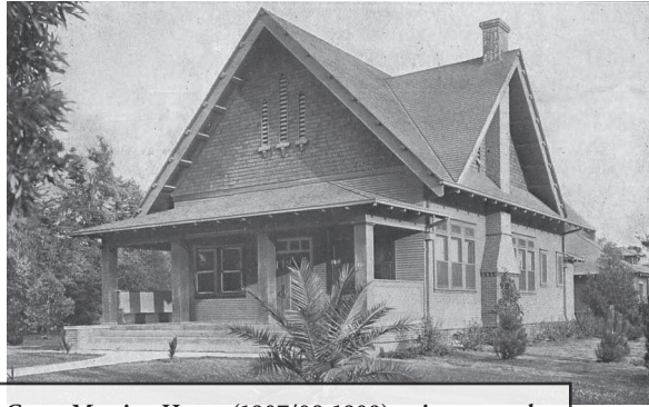
Figure 22. The Orange Grove Meeting House (1907/08-1909) as it appeared originally before construction of the fellowship room in 1918. Note the steeply pitched roofs and the resulting tall gables stressed by the deep roof eaves typical of the Craftsman bungalow. From a postcard mailed on January 12, 1914. Photo: Judson Emerick, from the original in the public domain
